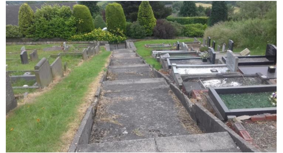
Photo 12: Top of flight of concrete steps looking down towards point C, black iron gates onto Taylor Lane 22/6/2017
