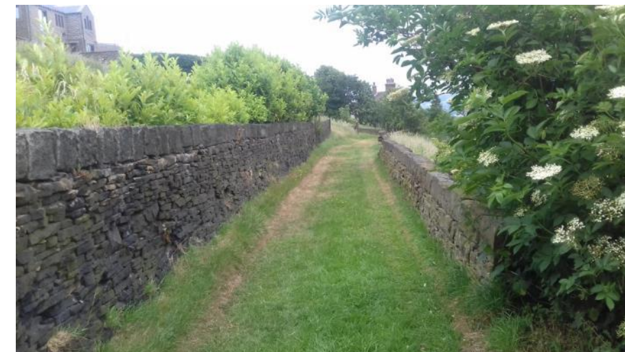
Photo 3: Walled wide grassy lane with vehicle tracks, 4 Vermont Close top left at BE 22/6/2017
